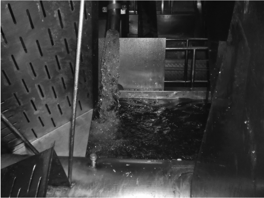
Figure 21.8 This photo shows the enormous amount of fresh, cold, chlorinated water being added to the exit end of the chiller in Chile. This made the water in the chiller extremely clean and low in organic material.
