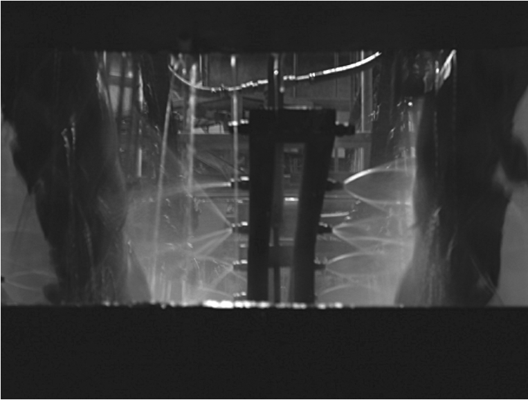
Figure 18.1 An improperly operating spray bar with nozzles plugged.
