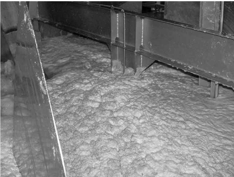
Figure 21.4 Another example of the exit of a chiller with water containing high levels of fat due to overscalding.
