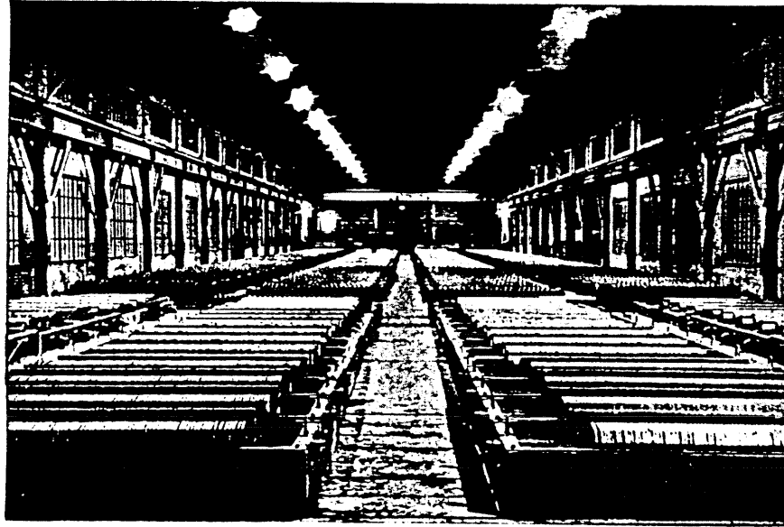
FIG. 4.—Night view of Betts tank house; dip washing tanks for corroded anodes in foreground.
