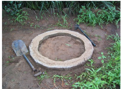
Figure 3-17: Completed ring beam
