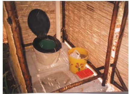
Figure 4-18: Inside a Fossa alterna that has been fitted with a pedestal
