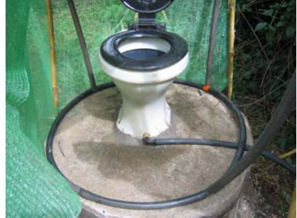
Figure 7-8: Urine-diverting pipe attached to base of pedestal
