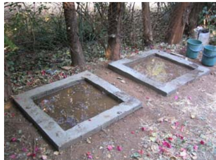
Figure 6-48: Cured ring beams
