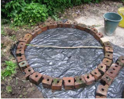
Figure 3-22: Circle of bricks 1.15m in diameter
