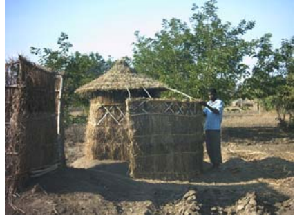
Figure 3-54: A functional and attractive structure
