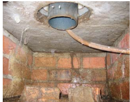
Figure 7-14: Urine pipe located below the slab
