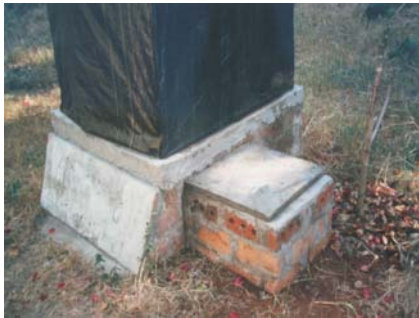
Figure 6-39: Side-vault for urine collection
