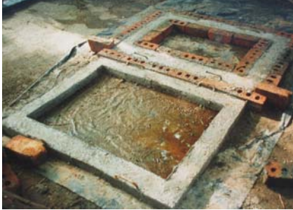
Figure 4-9: Ring beam mould using bricks
