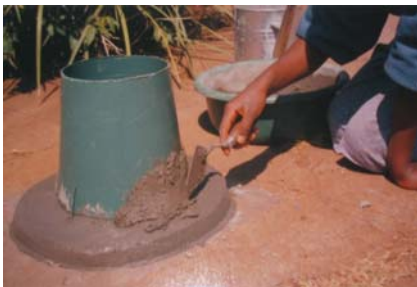
Figure 5-1: Construction of the very low cost pedestal
