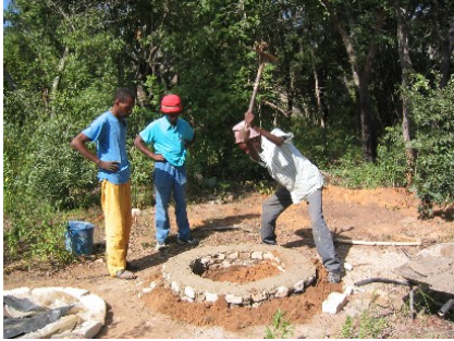
Figure 3-33: Digging the pit inside the brick ring beam
