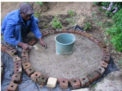
Figure 3-26: Wires added for reinforcement
