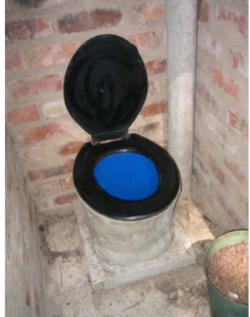
Figure 5-12: Completed low cost pedestal with plastic seat
