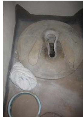
Figure 4-4: Inside of the permanent structure
