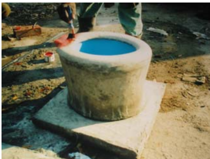
Figure 5-5: Painting the concrete pedestal
