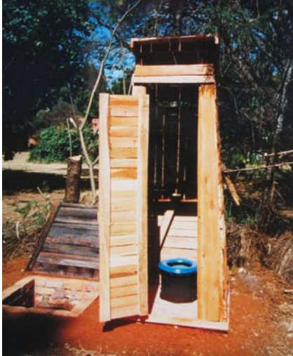
Figure 4-15: Fossa alterna using a wooden structure
