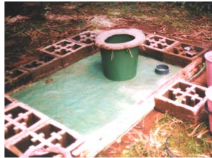
Figure 6-2: The brick mould for the toilet slab
