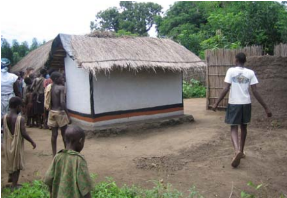
Figure 4-3: A permanent structure housing both pits
