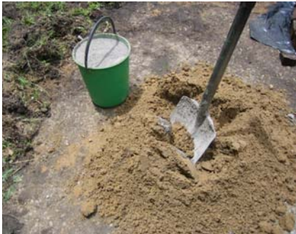
Figure 3-24: Mixing the cement and river sand
