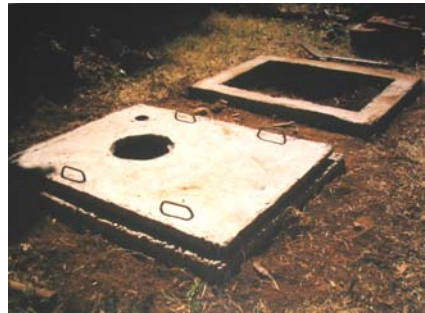
Figure 4-14: The completed pits for the double pit composting toilet
