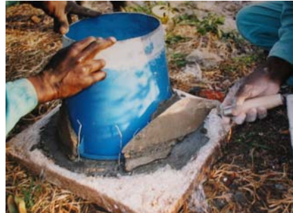
Figure 5-4: Building up the sides of the bucket
