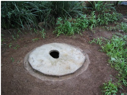
Figure 3-20: Toilet slab placed on ring beam
