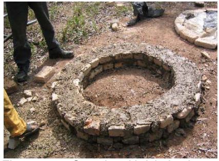
Figure 3-12: Completed brick ring beam
