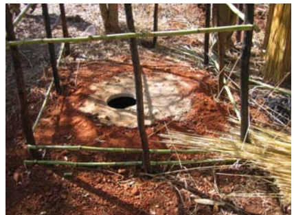
Figure 3-50: Gum poles, reeds and grass used to build the wall
