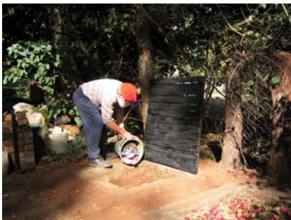
Figure 6-53: Emptying the bucket of faeces into the pit
