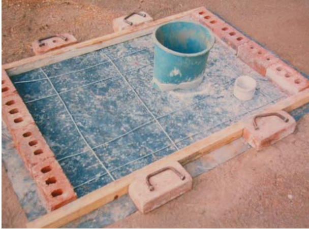
Figure 4-6: A slab mould made with bricks and wood
