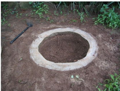
Figure 3-18: Digging of hole inside ring beam
