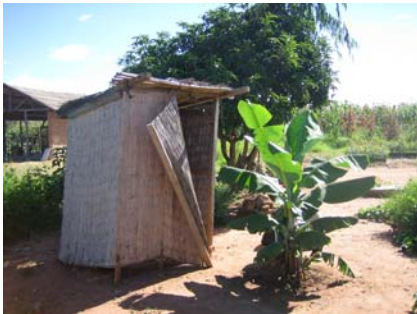
Figure 3-39: Toilet house built with local materials
