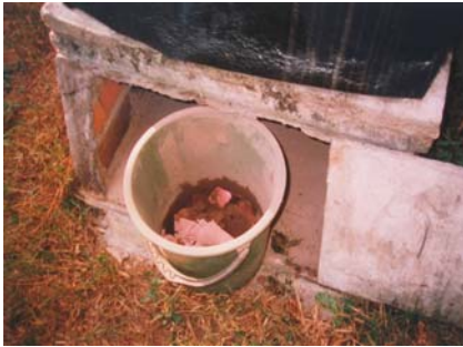
Figure 6-43: Removal of bucket of faeces
