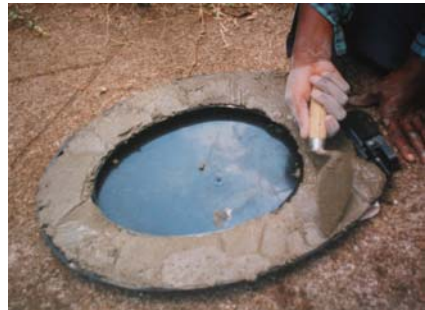
Figure 5-8: Plastic toilet seat filled with strong concrete
