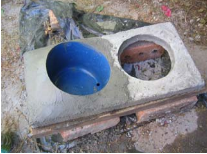
Figure 6-33: Top-view of a urine-diverting squat toilet
