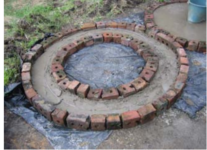
Figure 3-30: Concrete mix added to mould
