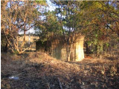
Figure 3-51: Completed toilet house
