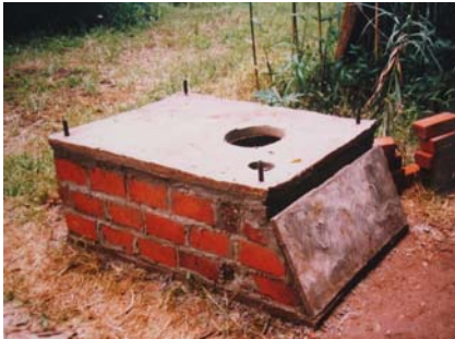
Figure 6-5: Fitting the vault access slab
