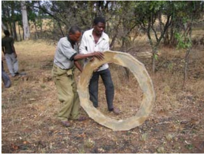
Figure 3-45: Moving the dry ring beam to a new site
