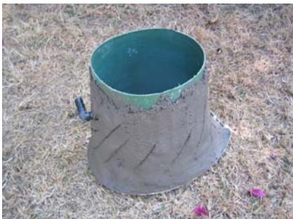
Figure 6-21: Upper-half of bucket covered in concrete
