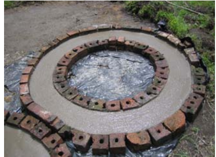
Figure 3-32: Remainder of concrete mix added and levelled-off
