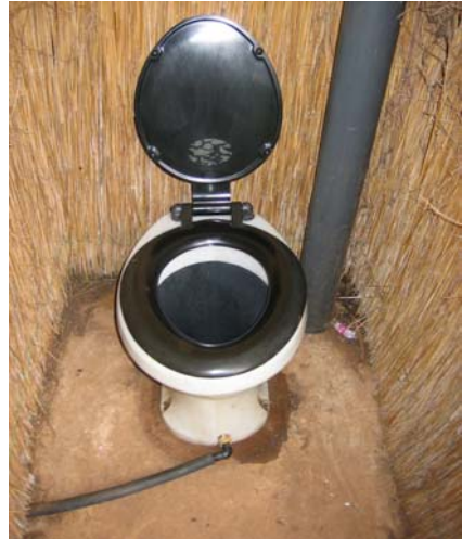
Figure 7-12: Fossa alterna upgraded with a urine-diverting pedestal
