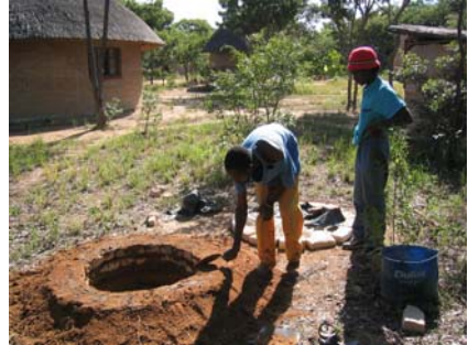
Figure 3-34: Packing soil around the brick ring beam
