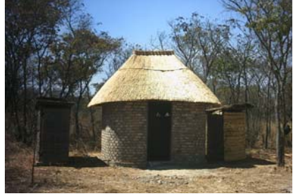
Figure 4-26: A Fossa alternata with a permanent brick and thatch structure
