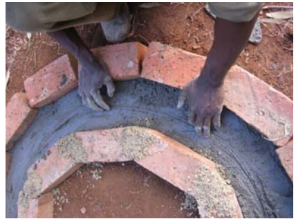
Figure 3-44: Addition of wire for reinforcement
