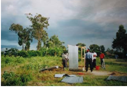
Figure 4-25: Construction of a portable structure for a Fossa alternata
