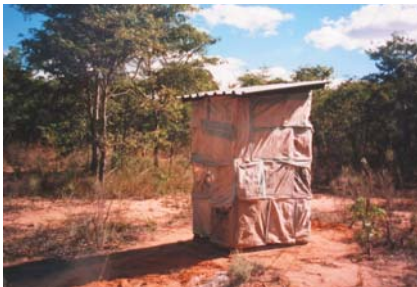
Figure 7-9: Arborloo built on a rectangular slab
