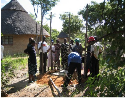
Figure 3-37: Using poles to build the toilet house
