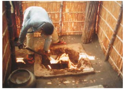
Figure 4-22: Excavating the humus from the pit
