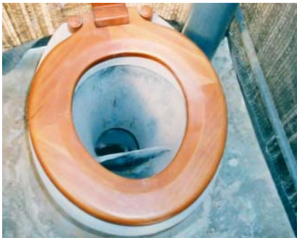
Figure 7-13: Urine-diverting pedestal mounted above the ground
