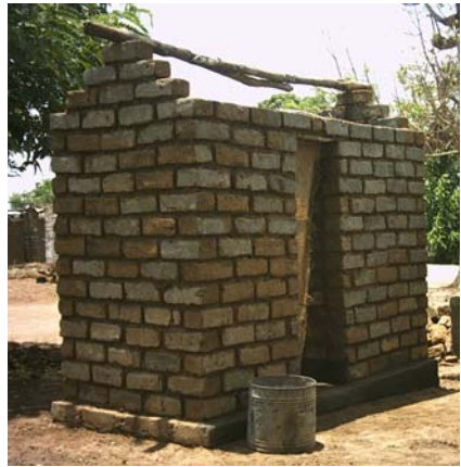
Figure 4-28: Brick double pit composting toilet
