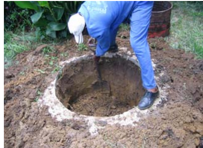
Figure 3-36: Digging the pit inside the concrete ring beam
