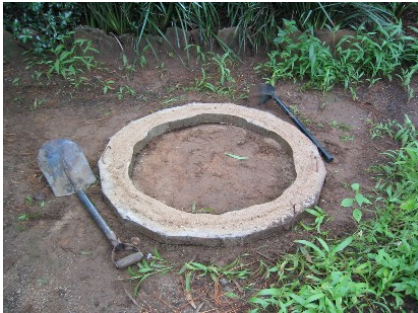
Figure 7-3: Ring beam laid on level ground
