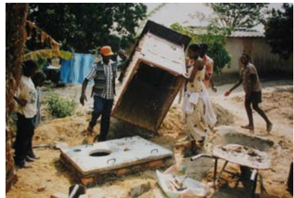
Figure 7-10: Fossa alterna built on a rectangular slab
