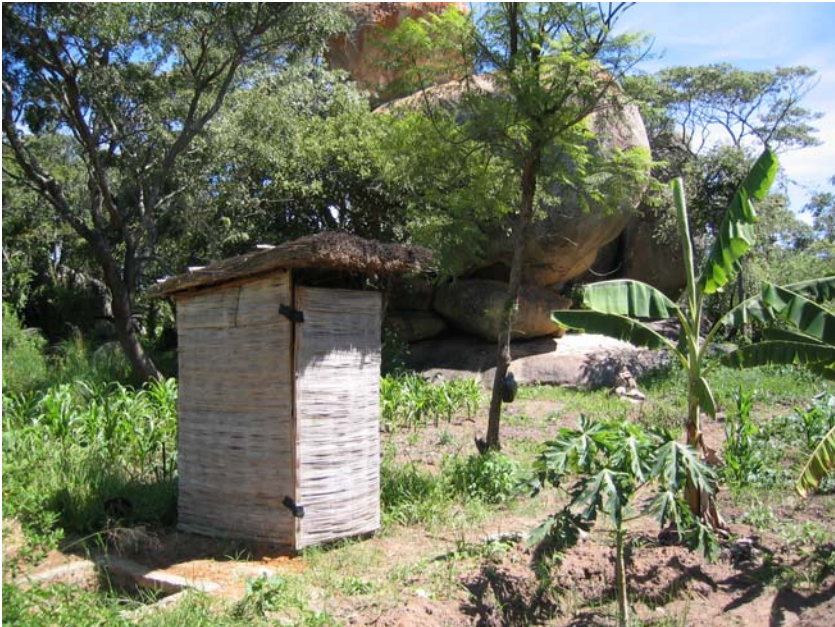
Figure 13-1: Eco-toilet in Ruwa, Zimbabwe
