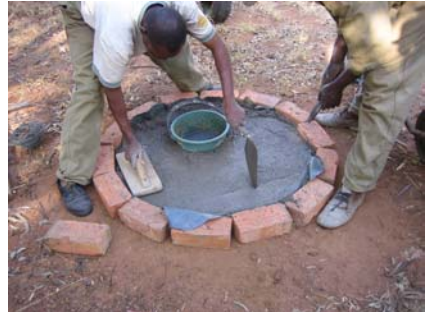
Figure 3-42: Levelling-off the concrete mix
