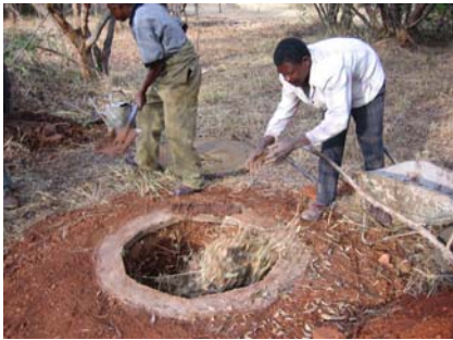
Figure 3-47: Addition of leaves to pit
