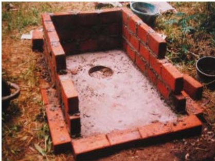
Figure 6-3: Building the vault using bricks on their edge
