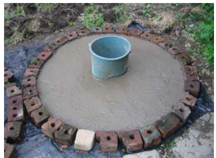
Figure 3-27: Remainder of concrete mix added and levelled-off
