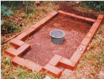
Figure 6-1: The brick mould for the base slab
