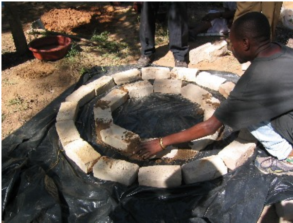
Figure 3-13: Brick mould on top of plastic sheet
