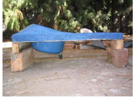
Figure 6-34: Side-view of a urine-diverting squat toilet
