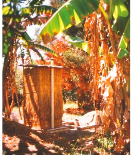
Figure 4-16: Fossa alterna with grass walls
