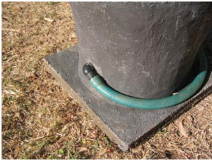
Figure 6-27: Urine outlet pipe attached
