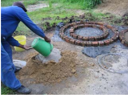
Figure 3-29: Mixing the cement and river sand
