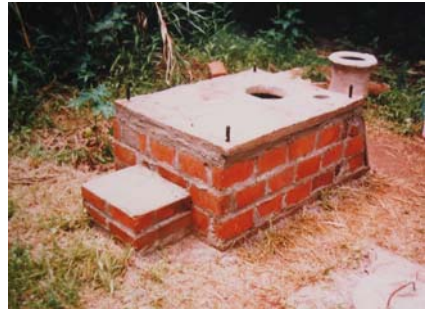
Figure 6-6: Front view of the vault with the toilet slab placed on top
