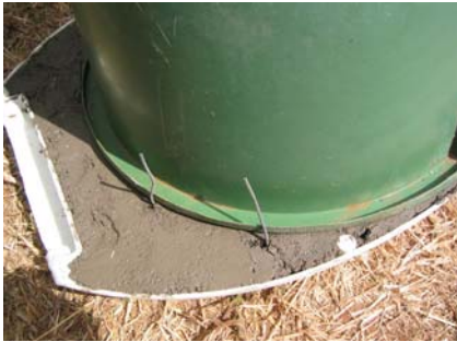
Figure 6-19: Bent wire added around the bucket
