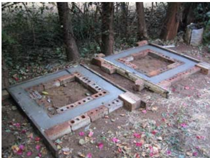
Figure 6-47: Casting ring beams
