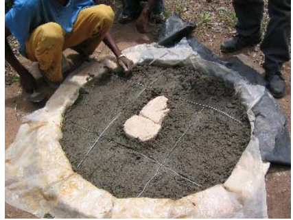
Figure 3-8: Cement and reinforcing wires in mould
