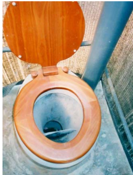
Figure 6-36: Top-view of the a urine-diverting pedestal
