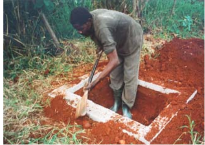
Figure 4-10: Digging the pit for the Fossa alterna
