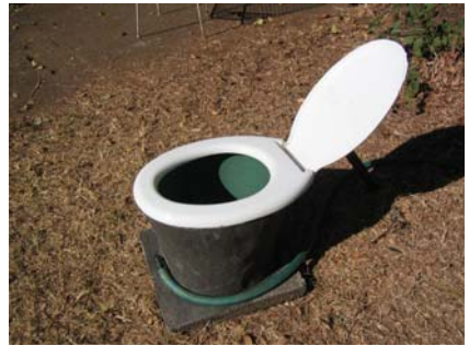
Figure 6-28: Outlet pipe led to the back of the toilet
