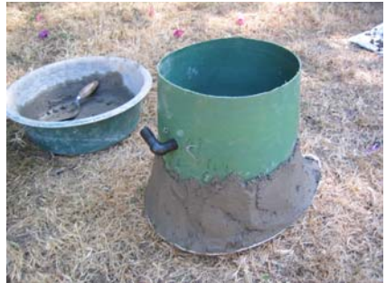
Figure 6-20: Concrete added half-way up the bucket
