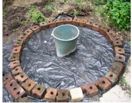
Figure 3-23: Shaped bucket to make the squat hole
