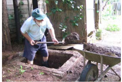
Figure 10-14: Digging-out the toilet compost
