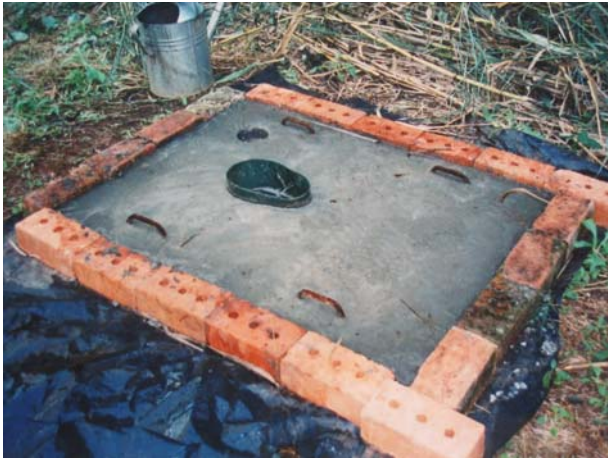
Figure 4-7: The completed slab inside the mould
