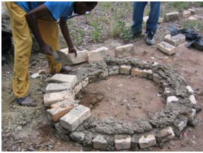
Figure 3-11: Adding the second layer of bricks with anthill mortar
