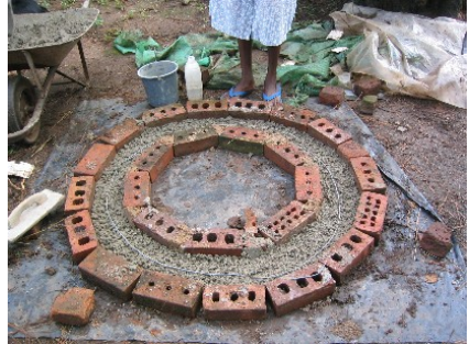
Figure 3-15: Cement and wire reinforcement added to mould
