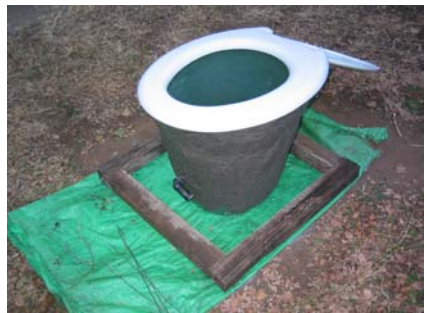
Figure 6-22: Bucket and seat turned over and placed into base mould
