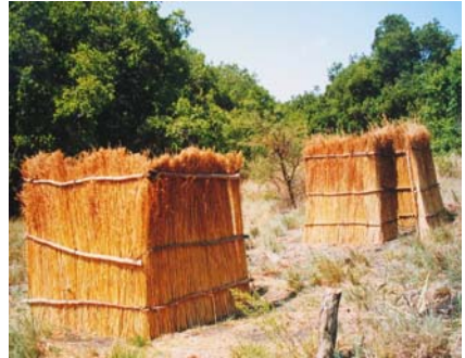
Figure 3-38: Toilet houses without a roof
