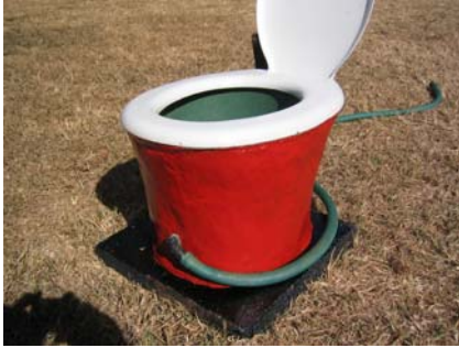
Figure 6-29: Painting the pedestal
