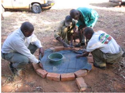
Figure 3-41: Laying down reinforcement wires
