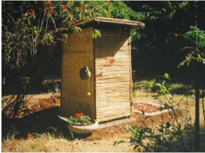
Figure 4-1: A portable structure using poles and reeds
