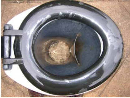
Figure 7-1: Urine-diverting pedestal fitted to a Fossa alterna system
