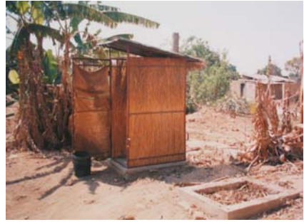
Figure 4-2: A portable structure using a steel frame
