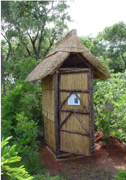
Figure 3-1: Simple compost toilet built on rectangular slab
