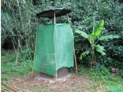
Figure 7-7: Structure around upgraded toilet
