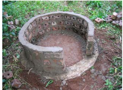
Figure 7-4: Brick wall built-up on ring beam
