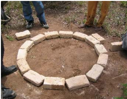
Figure 3-5: Ring of bricks for the mould
