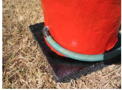
Figure 6-30: Close-up of the base of the pedestal
