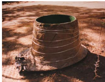
Figure 5-10: Concrete reinforcement added around first layer of concrete
