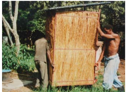
Figure 3-58: A portable structure built using a frame of steel
