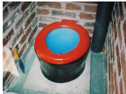
Figure 5-6: Finished concrete pedestal
