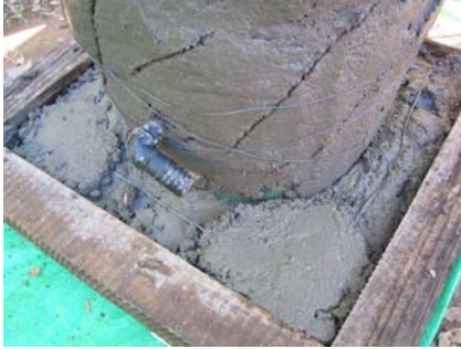
Figure 6-23: Wire added for reinforcement
