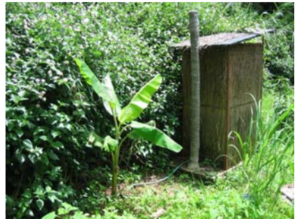
Figure 6-32: Exterior of toilet house with urine-diverting toilet
