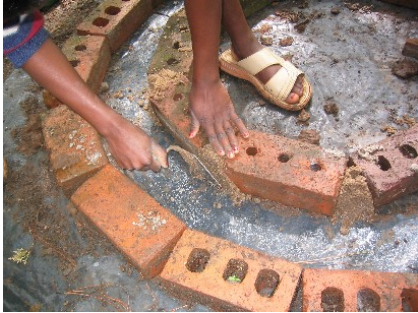
Figure 3-14: Filling the spaces in the inner brick mould
