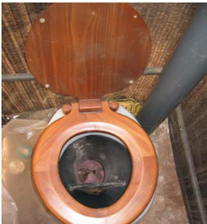
Figure 6-57: Cleaned urine-diverting toilet
