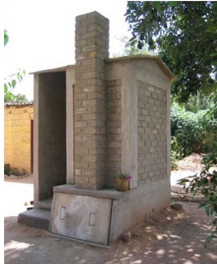
Figure 6-42: A brick single-vault urine-diverting toilet
