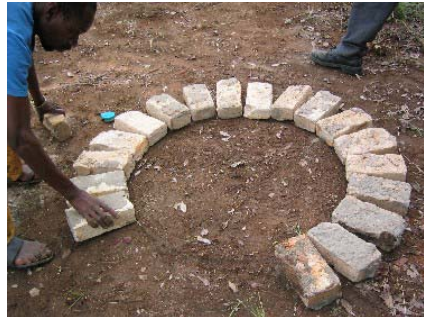
Figure 3-10: Forming the brick ring beam
