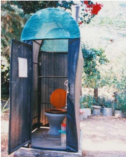
Figure 6-41: Superstructure made of polyethylene pipes covered with a plastic cloth
