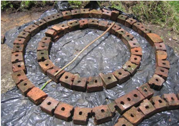
Figure 3-28: Two brick circles for ring beam mould
