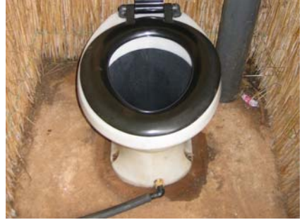
Figure 7-2: Urine off-take fitted above the base of the pedestal
