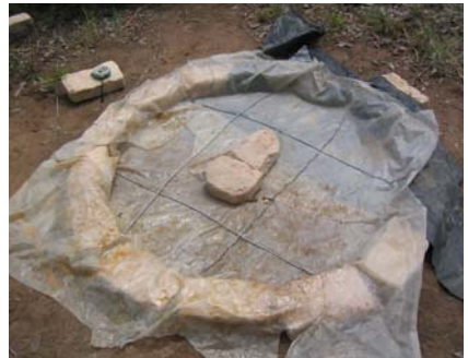
Figure 3-6: Sheet of plastic laid in the mould
