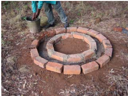
Figure 3-43: Ring beam mould using bricks
