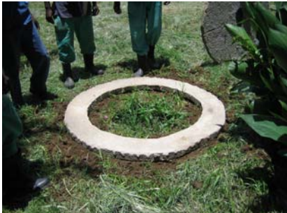
Figure 3-35: Placement of the concrete ring beam
