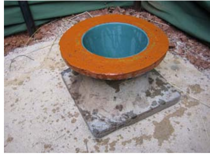
Figure 3-52: Low-cost pedestal on top of slab
