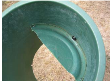
Figure 6-14: Inside view of the fitted pipe bend
