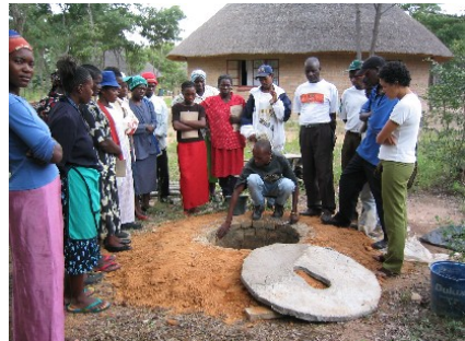
Figure 3-21: Trainees at Kufunda village
