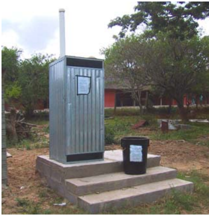
Figure 4-27: Fossa alternata with a metal structure
