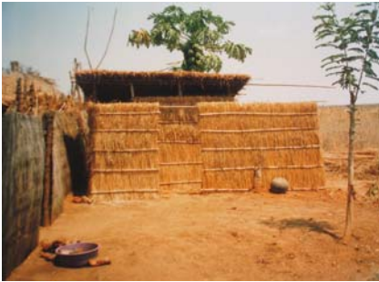
Figure 4-21: Fossa alterna with a permanent structure
