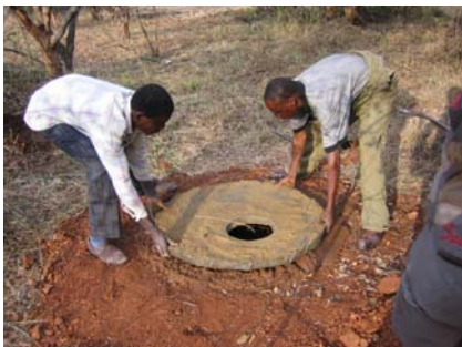
Figure 3-49: Slab placed over ring beam
