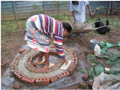
Figure 3-16: Levelling off the concrete
