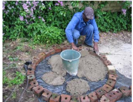
Figure 3-25: Adding the cement and sand mix to the mould
