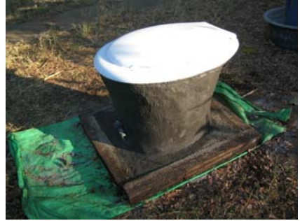
Figure 6-24: Completed pedestal curing
