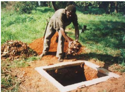
Figure 4-11: Adding leaves to the Fossa alterna pit
