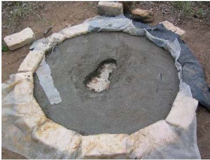
Figure 3-9: Mould after removal of squat hole insert
