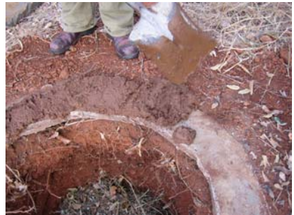
Figure 3-48: Anthill mortar packed around ring beam
