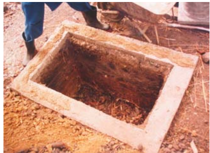
Figure 4-12: Completed Fossa alterna pit
