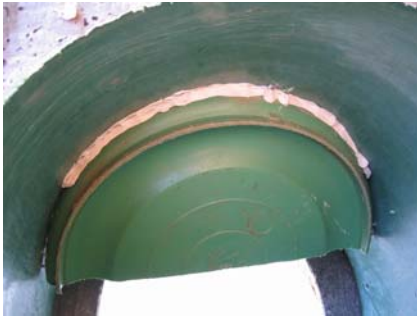
Figure 6-25: Sealing the urine diverter against the bucket wall
