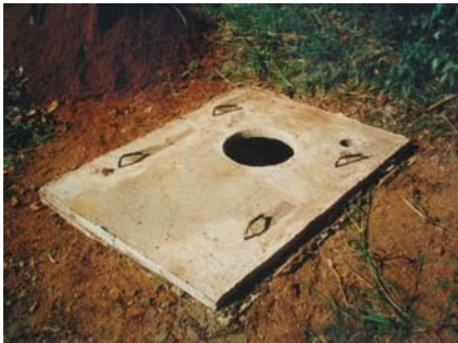
Figure 4-13: Addition of the concrete slab
