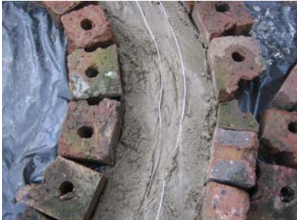
Figure 3-31: Wire reinforcement added
