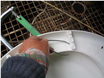
Figure 6-15: Using a hot wire to make a hole through the plastic toilet seat ribs
