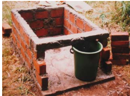
Figure 6-4: Testing the height of the vault access
