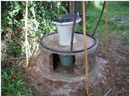
Figure 7-5: Slab and pedestal fitted on built-up base
