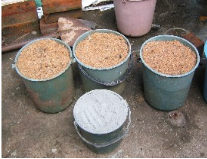
Figure 3-7: Measuring cement and river sand
