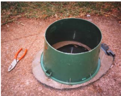
Figure 5-9: Plastic bucket placed over toilet seat
