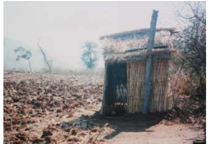
Figure 3-56: Another style of structure with a ventilation pipe
