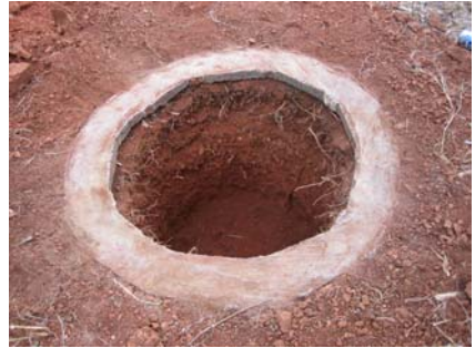
Figure 3-46: Pit dug inside ring beam
