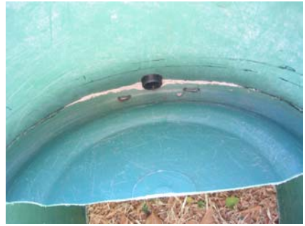
Figure 6-26: Sealing the top side of the urine diverter
