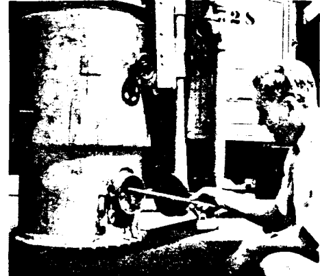
Chunks of charcoal-like ash are removed from the generator daily through a cleanout door
