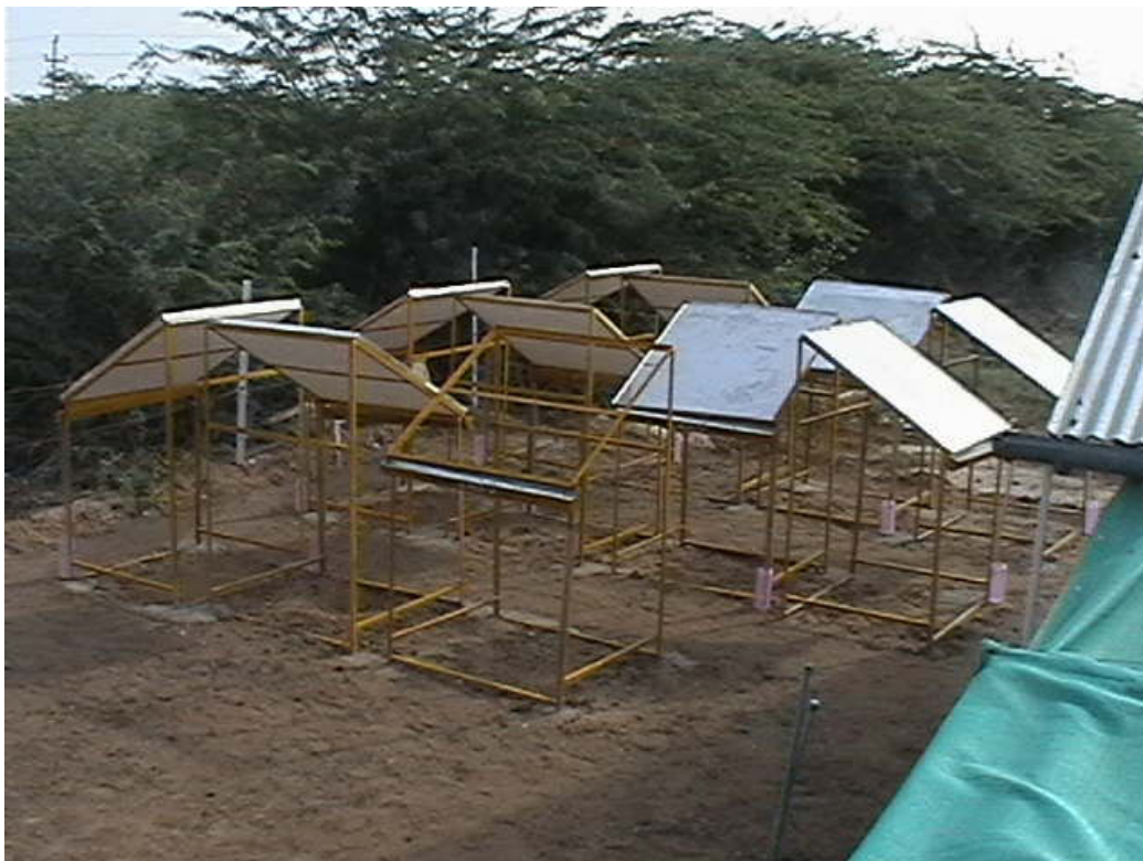
Figure 2. Condensers Test site at Kothara
