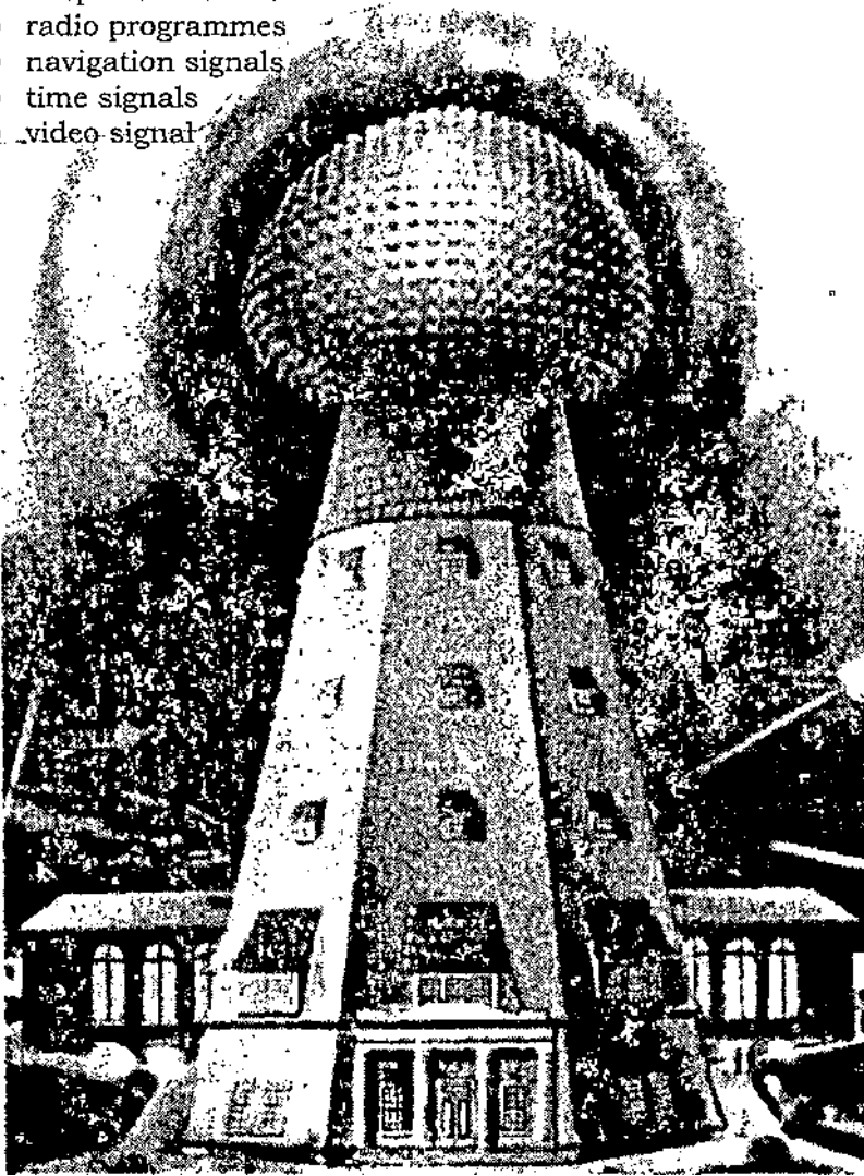
Fig. 9.10: The planned transmitter Wardencliff of Tesla on Long Island, 7.5 MW (1902).
