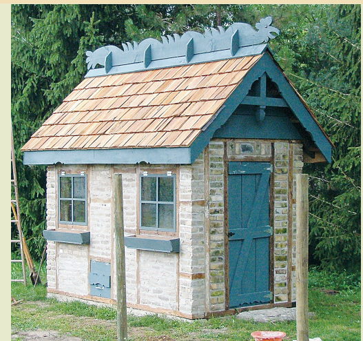
Using a German technique called fachwerk, the owners first constructed a timber framework and then filled panels with brick and mortar.
