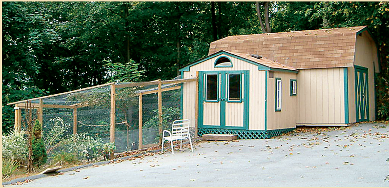
Affectionately dubbed the Hensington Palace, this coop was made using a prefab garden shelter that was attached to an existing garage. The windows were purchased at a surplus store and added to it.
