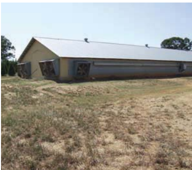
Figure 3-2 Poultry house with tunnel ventilation. Photo by Sarah Kane, Courtesy of Cabe Brothers Farm.
