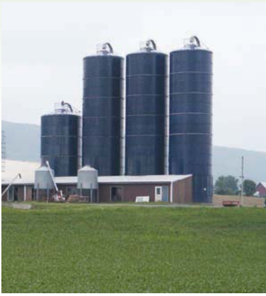
Figure 18-7 Conventional silos used for storing grain and other feeds. Courtesy of Harvestore–Engineered Storage Products Co.
