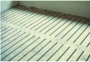
Figure 24-1 Slotted floors help in the handling and removal of manure in swine facilities. Courtesy of Dr. Robert Dove, University of Georgia.
