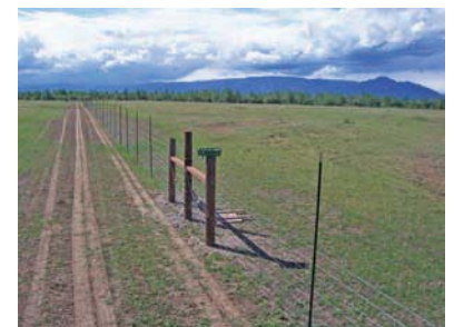
Figure 48-5 This game fence in Alaska will be 8 feet high when completed. Courtesy of Alaska Interior Game Ranch, Inc.
