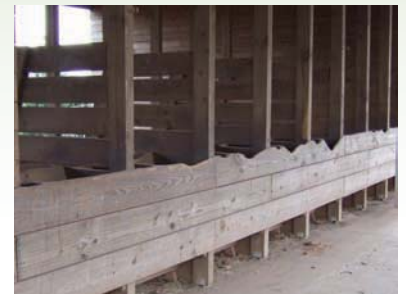
Figure 31-41 Stall panels worn down by cribbing horses. Photo by Dr. Frank Flanders.
