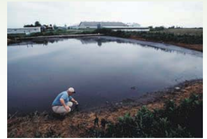
Figure 4-8 This hog operation utilizes a filtering system that consists of a series of hillside terraces that form constructed wetlands that also use bacteria to purify the wastewater. Courtesy of USDA Natural Resources Conservation Service. Photo by Tim McCabe.
