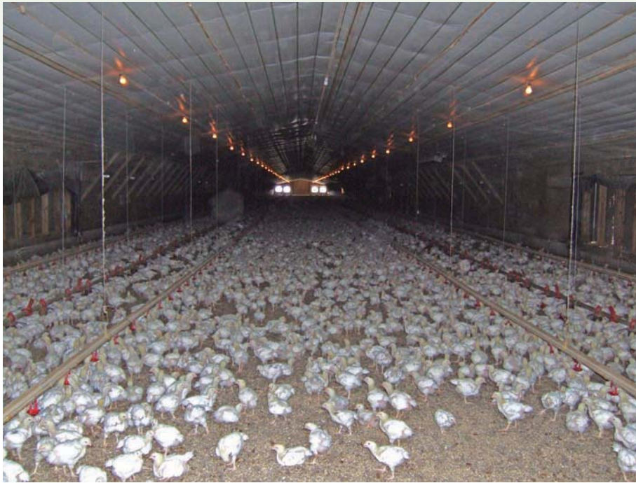
Figure 3-3 Tunnel vents in chicken houses help to circulate and cool the air and reduce the danger from the buildup of toxic gases. Photo by Sarah Kane, Courtesy of Cabe Brothers Farm.
