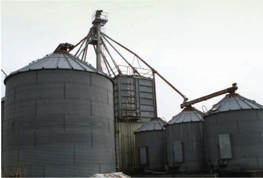
Figure 18-9 Metal storage bins are used to store grain and protein. Photo by Dr. Frank Flanders.
