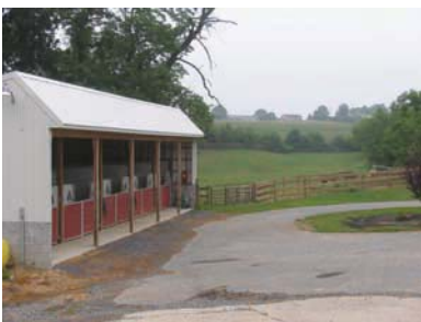
Figure 32-20 A horse barn with 12 × 12 feet box stalls and a covered way in front of the stalls. Photo by Dr. Jennie Simpson Osborne.
