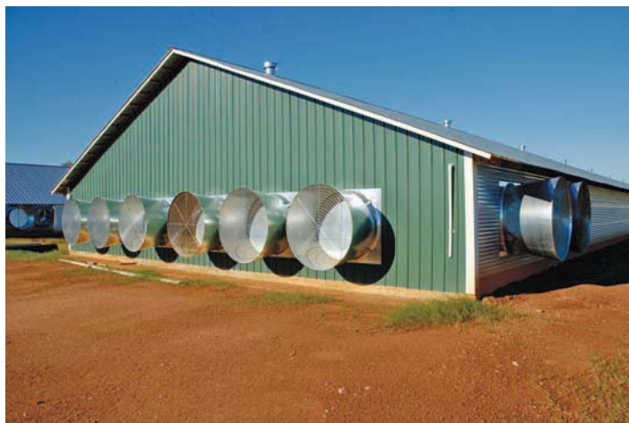
Figure 36-12 Exhaust fans attached to one end of a tunnel-ventilated poultry house pull air through cooling pads down the length of the facility. Courtesy of Chore-Time Poultry Production Systems, Milford, Indiana.
