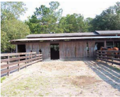
Figure 32-19 A small horse barn with space for feed, bedding, tack storage, and a runout paddock for each horse. Notice the hole in the boards where horses have chewed because of boredom. Photo by Victoria Churchill.
