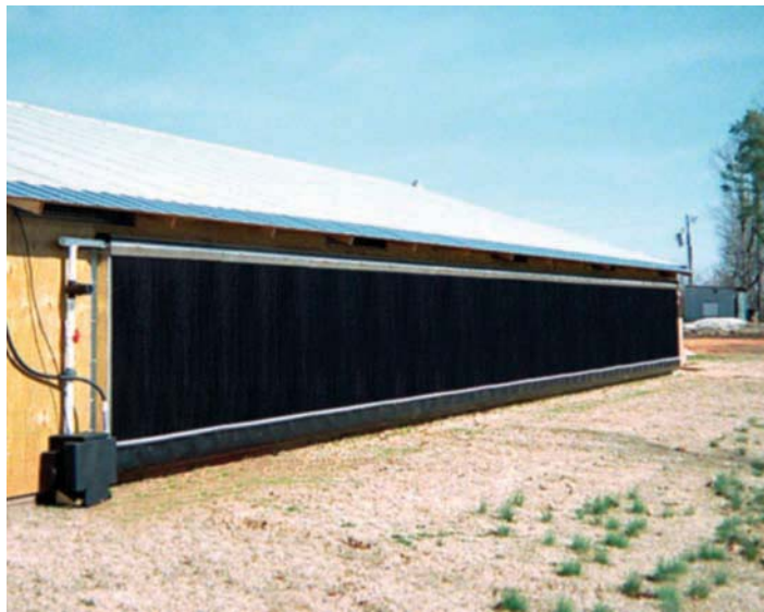
Figure 36-11 In tunnel-ventilated houses, cool cells (wet pads) are attached to one end of the house. Air pulled into the house by fans is cooled through the process of evaporation. Courtesy of Chore-Time Poultry Production Systems, Milford, Indiana.
