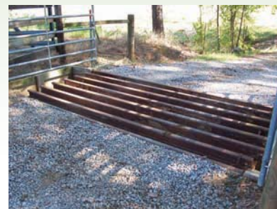
Figure 18-11 A cattle guard saves time in opening and closing gates. Photo by Victoria Churchill.
