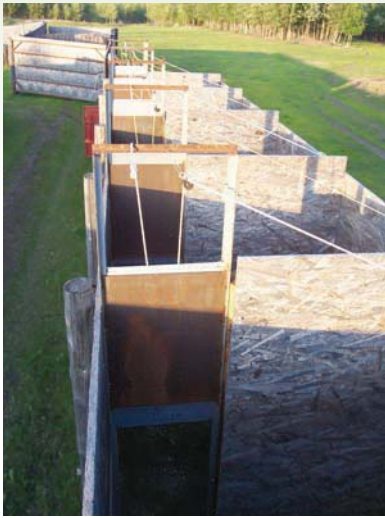
Figure 48-6 A running alley is used to move bison from the catch pens to the crowding area. Note the sturdy construction, solid panels, and 8-foot-high walls. Courtesy of Alaska Interior Game Ranch, Inc.
