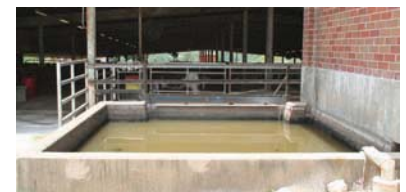
Figure 45-14 Gray water (waste water from milking, cleaning, etc.) is sometimes collected and used to flush free stall barns. Note the metal gate on this collection tank. Photo by Dr. Frank Flanders.
