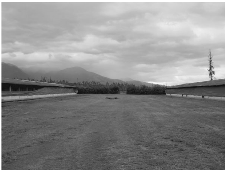
Fig. 5.3. Wide spacing between poultry houses.
