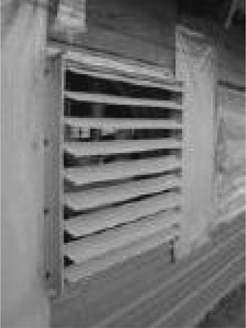
Fig. 5.29. Exterior shutter fan.
