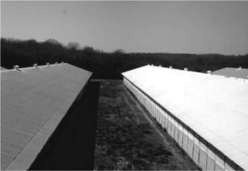
Fig. 5.10. Reflective roof coating.
