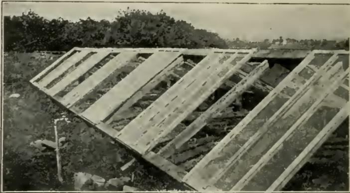
Fig. 19. A span-roof coldframe, or cold forcing-house.
