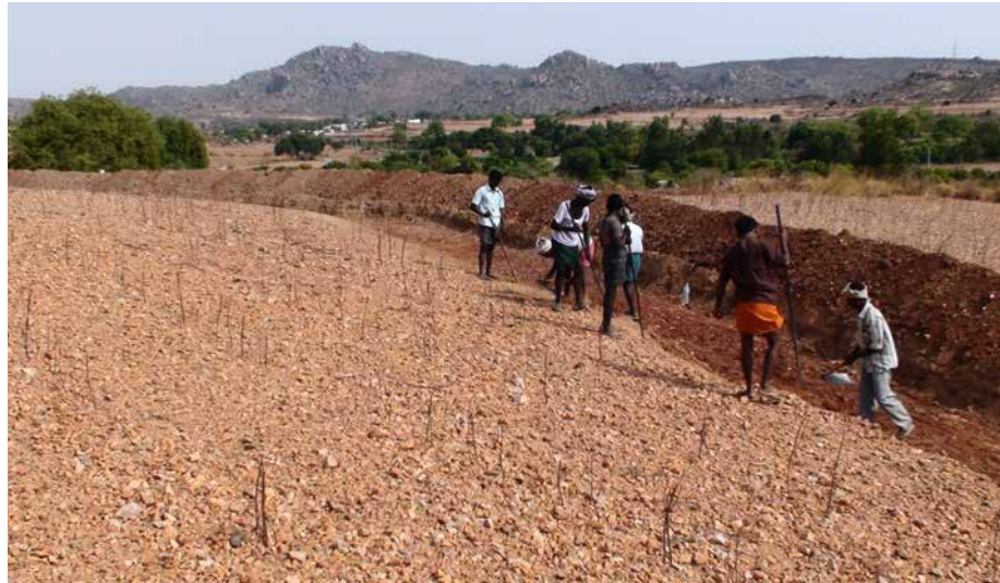
FIGURE 7.4. Workers groom the edges of the swale, using pikes to break through the hard soils.
