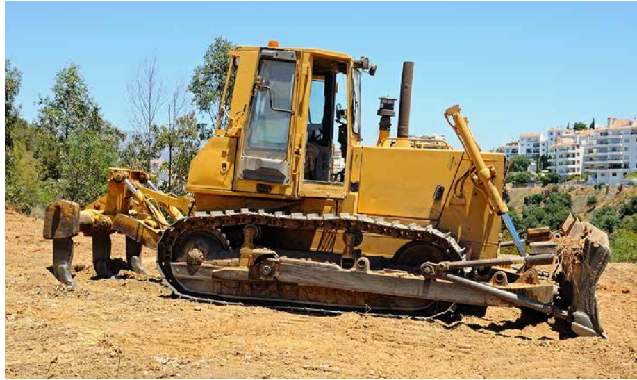
FIGURE 5.1. A bulldozer with VPAT blade (with straight blade attached) and rippers attached on the rear.
