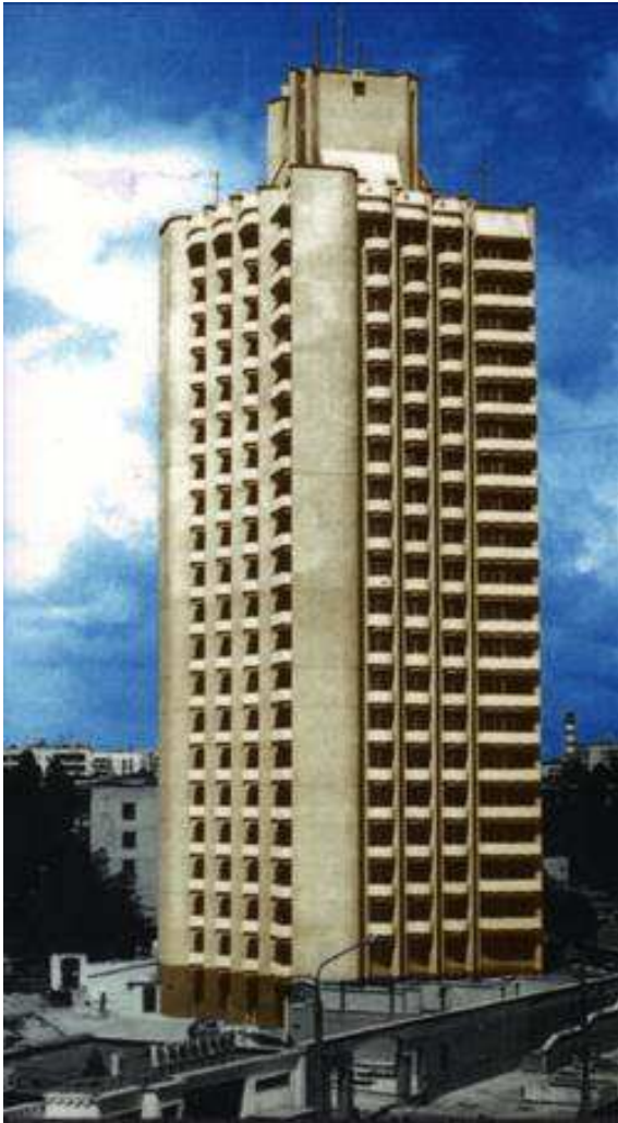
Fig.5. The first residential house made from alkali-activated cement concrete (Lipetsk, Russian Federation).
