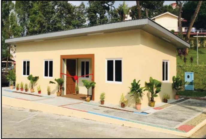
FIGURE 6.9 Geopolymer concrete house (first cement-free concrete house in Malaysia in Universiti Malaya campus for bus drivers).
