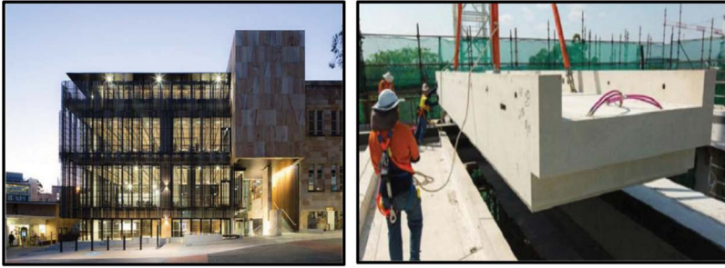
FIGURE 6.7 (a) Three-Storey Queensland's University GCI Building using structural GPC and (b) precast FA/slag-based GPC floor panel parts [26].
