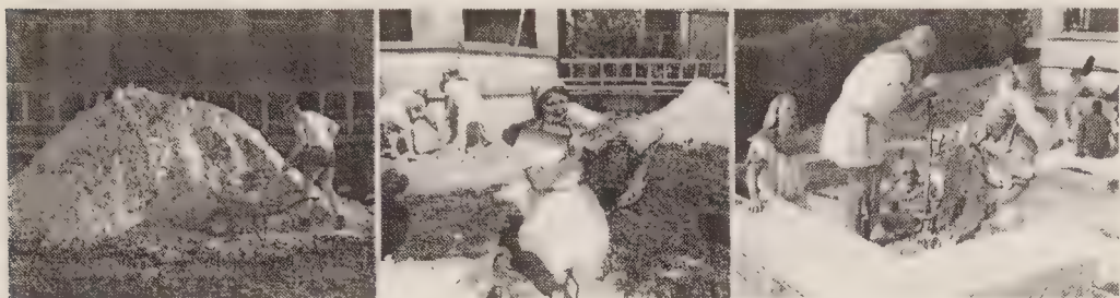
Figure 10.4: Fabrication stages : 1. the bulk of 14 tonnes of limestone. 2. transport with basket. 3. the packing with a rammer.
