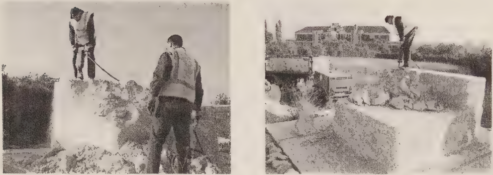
Figure 10.18: The construction being demolished with a pneumatic drill one year later.
