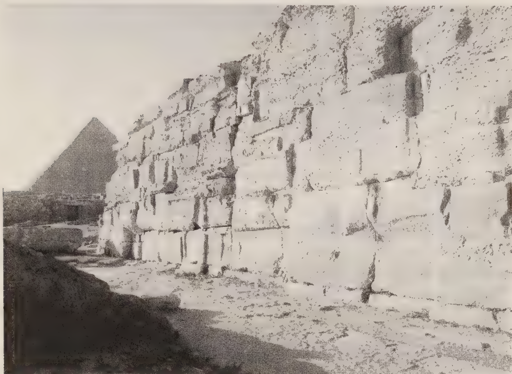
Figure A.38: Stage 17, Chephren Valley Temple (south side), limestone surface represents the negative face of the granite claddings (1984).
