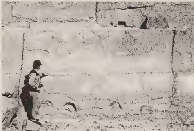
Figure A.18: Stage 7, Chephren Pyramid, south-east. Blocks showing curved jointing. (1984).
