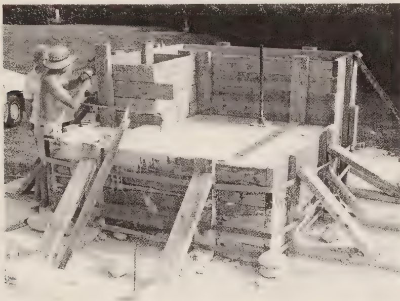
Figure 10.5: Mould made from small reusable wooden planks.
