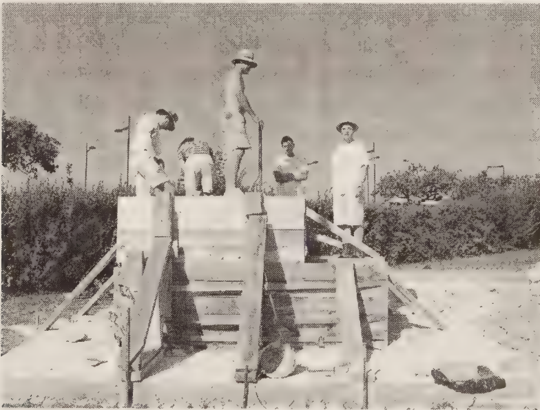
Figure 10.11: A team of five to make several blocks at day.
