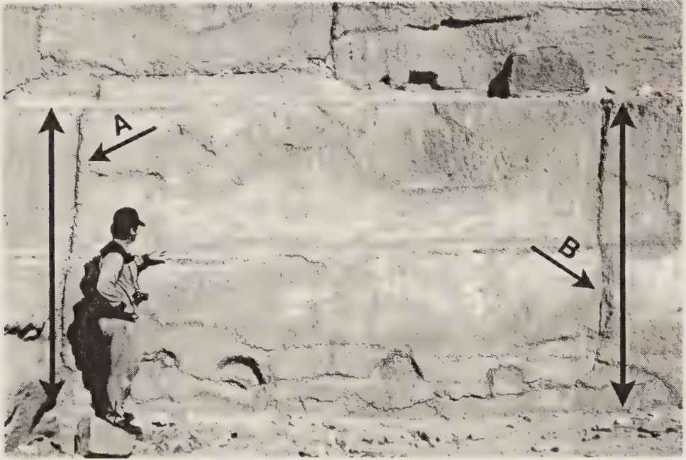
Figure 2.1: Blocks with vertical curved joints (A) (1984).
