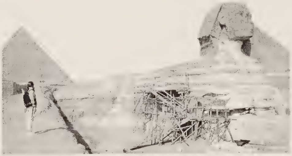
Figure 20.4: The body of the Sphinx was sculpted in the soft severely eroded limestone layer (1988).
