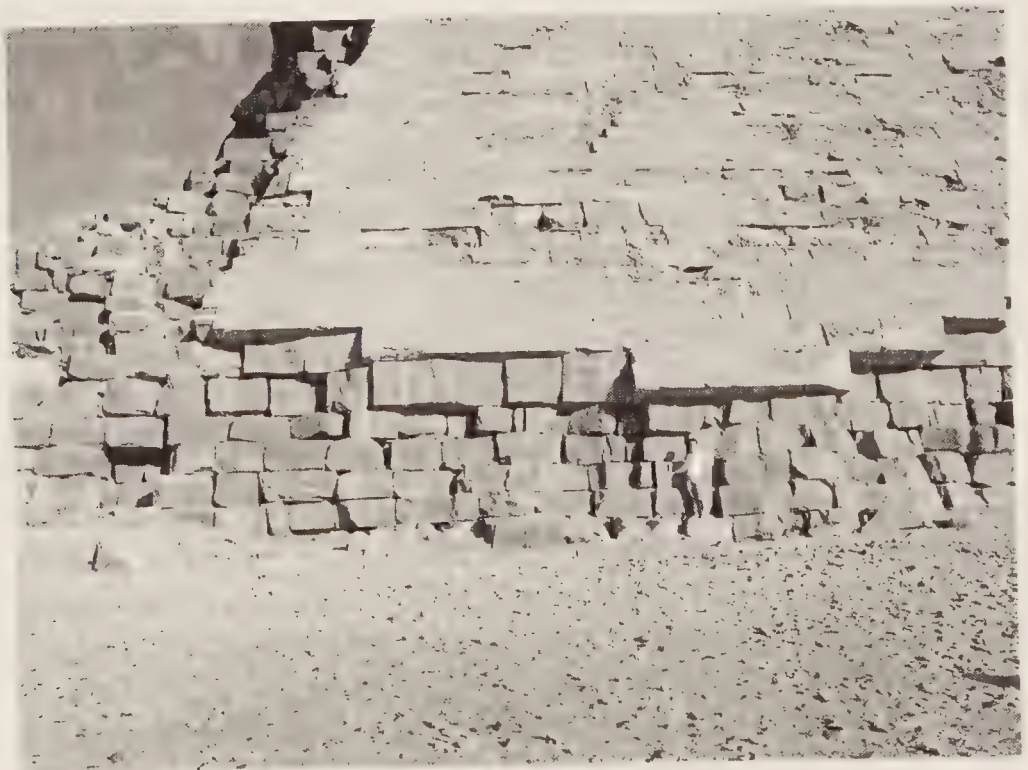
Figure 19.9: Bent Pyramid, succession of thickness from 0.50 metres (scale) to 0.80 metres (2003).
