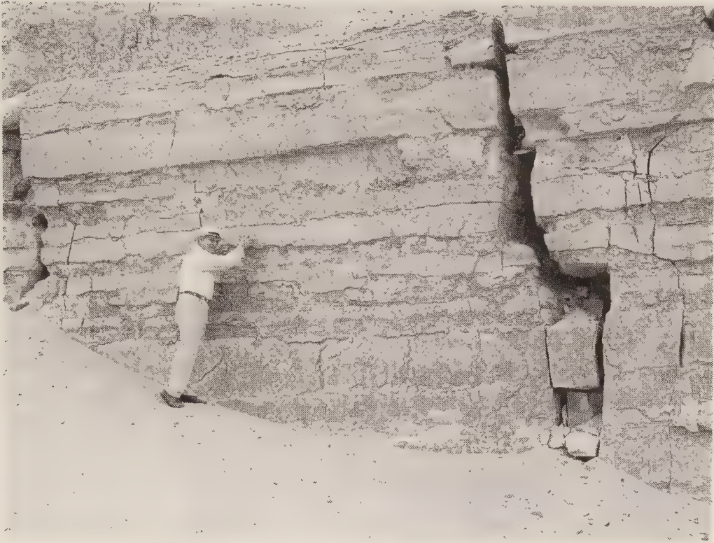
Figure 26.3: Alternating layers of hard and soft limestone at Saqqarah (2003).
