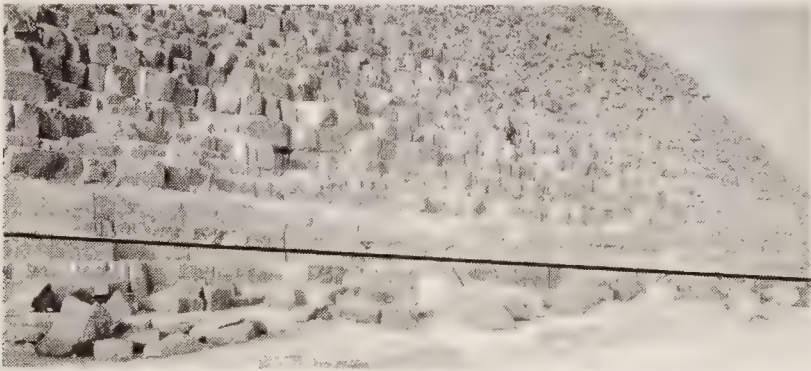
Figure A.16: Stage 6, middle of the south side of Chephren Pyramid. Inclined bedrock, thick line (1984).
