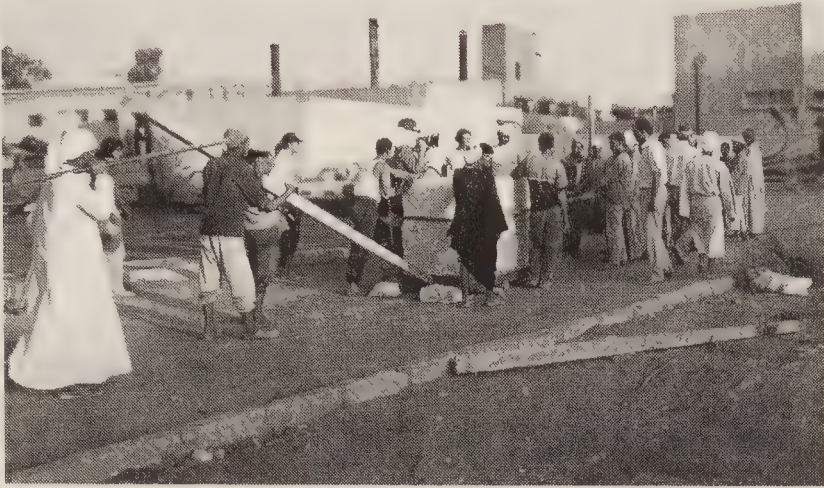
Figure 3.7: The experiment carried out by the NOVA team; pulling a large stone on rollers is only possible on a hard, flat surface such as a modern tarmac road. It does not work on sand (1991).
